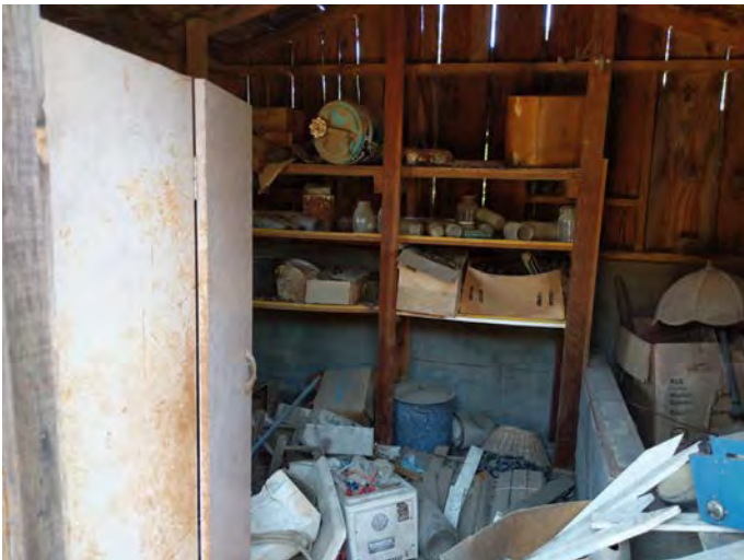
Typical interior views of the outbuildings
