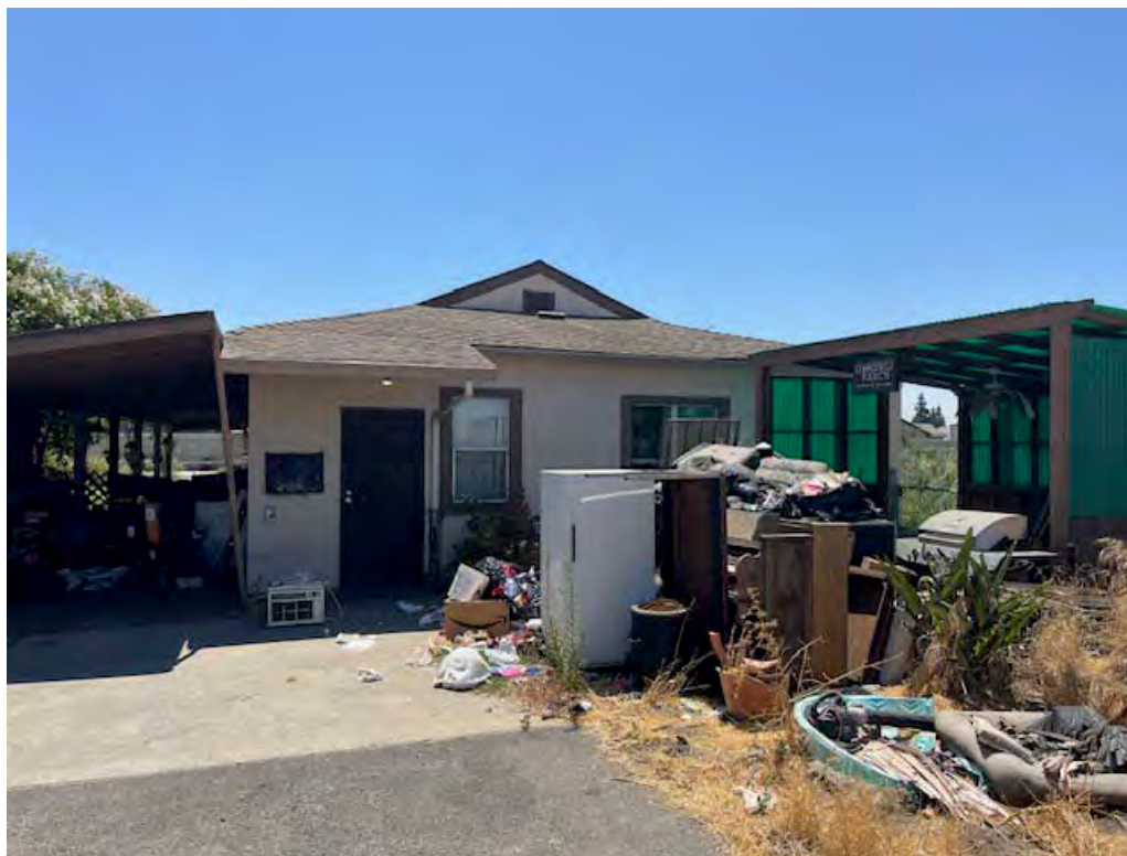
Residence looking south, 8/5/2024 note patio roof (left) is an addition.
