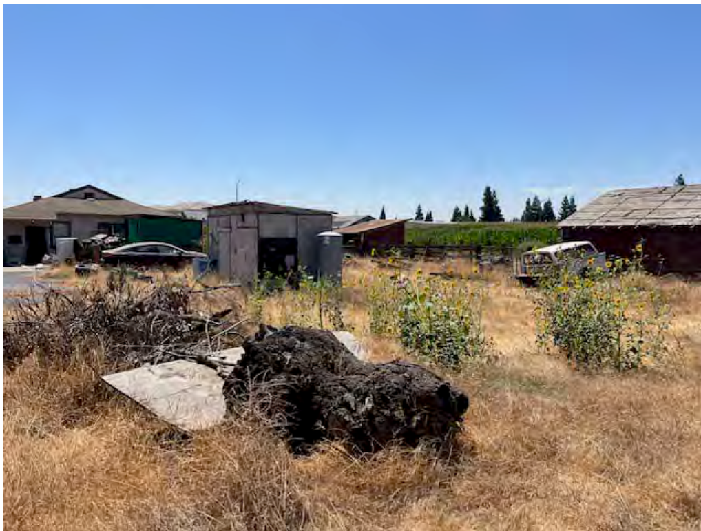
Looking SW, residence on left and 3 sheds, 8/5/2024
