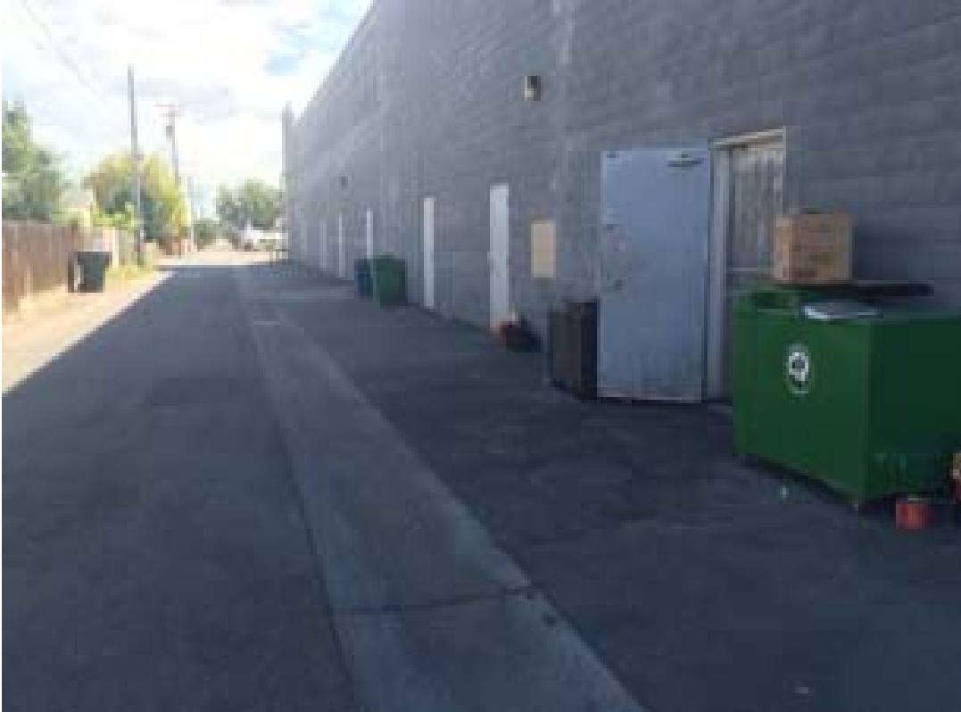
Used oil storage and grease interceptor on east side of building.
