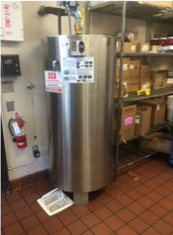
Used oil storage
