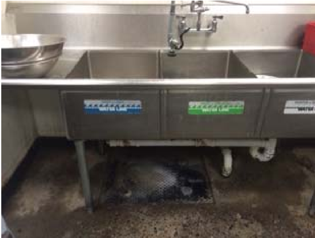
Under the sink trap
