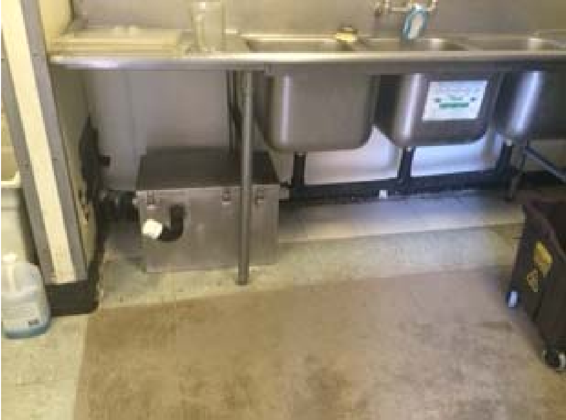
Under the sink trap
