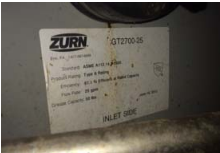
Under the sink trap
