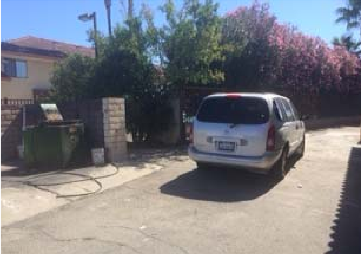
Interceptor on East side of building
