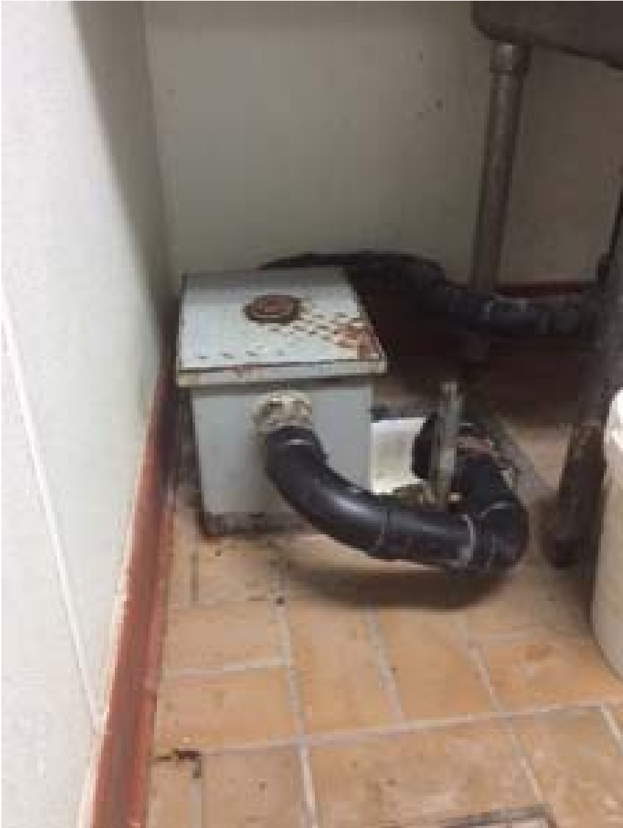
Small under the sink trap
