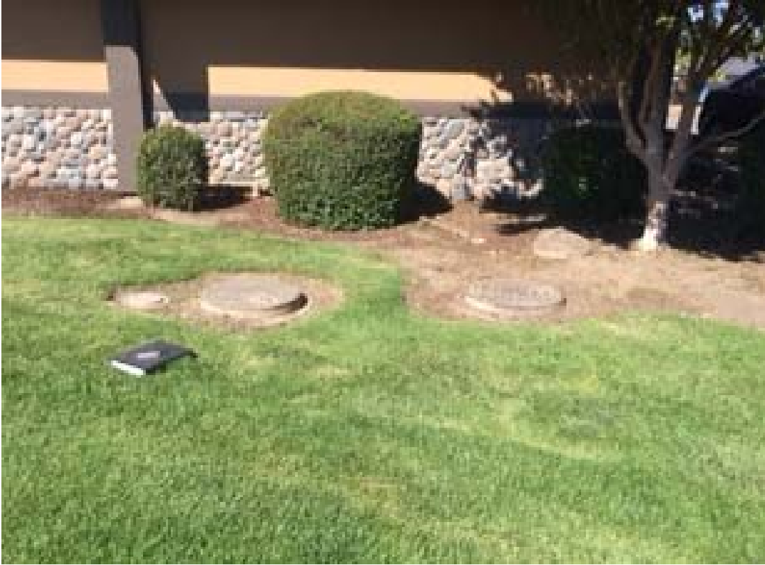
Interceptor in south landscaping of restaurant
