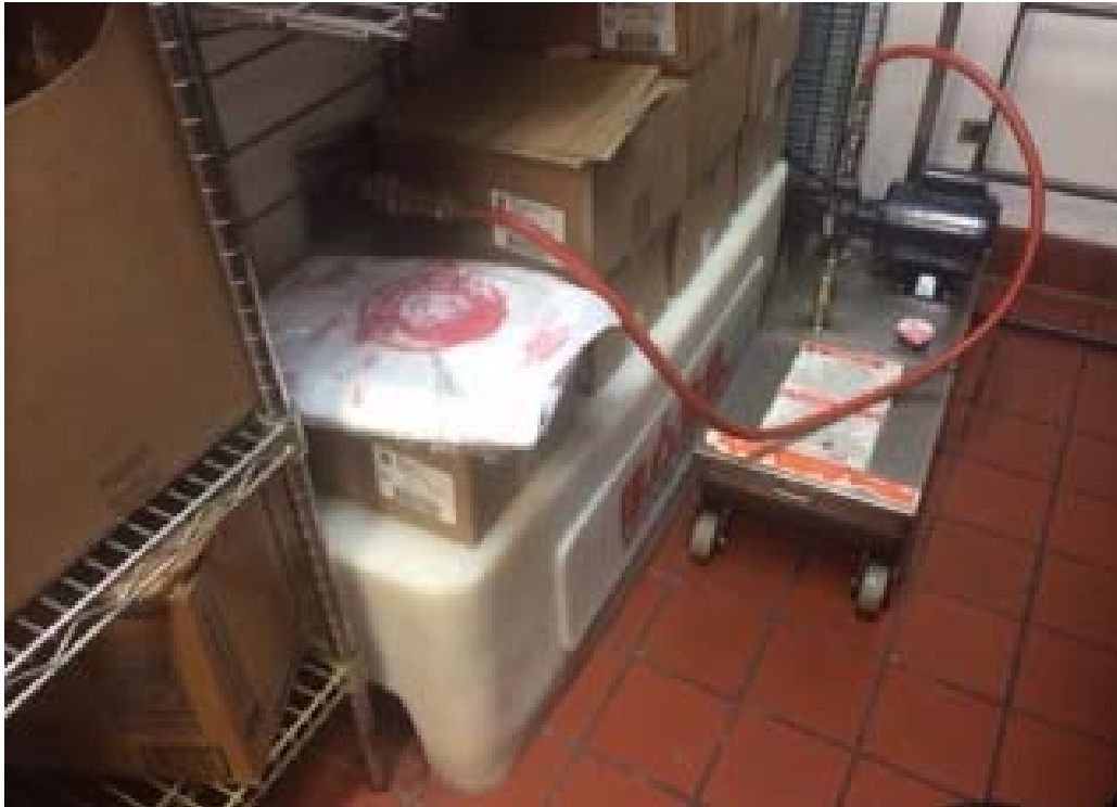
Used oil storage
