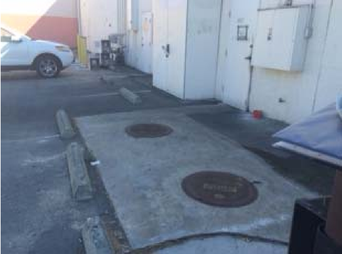
Interceptor behind restaurant
