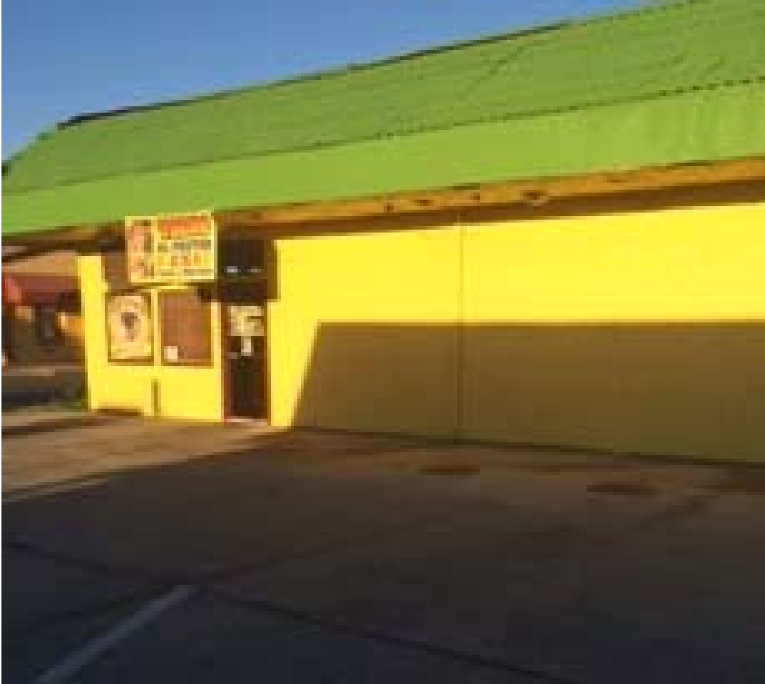
Interceptor in parking lot.
