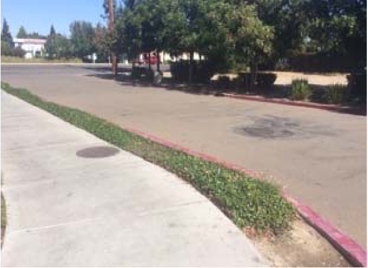
Large Interceptor in parking entrance
