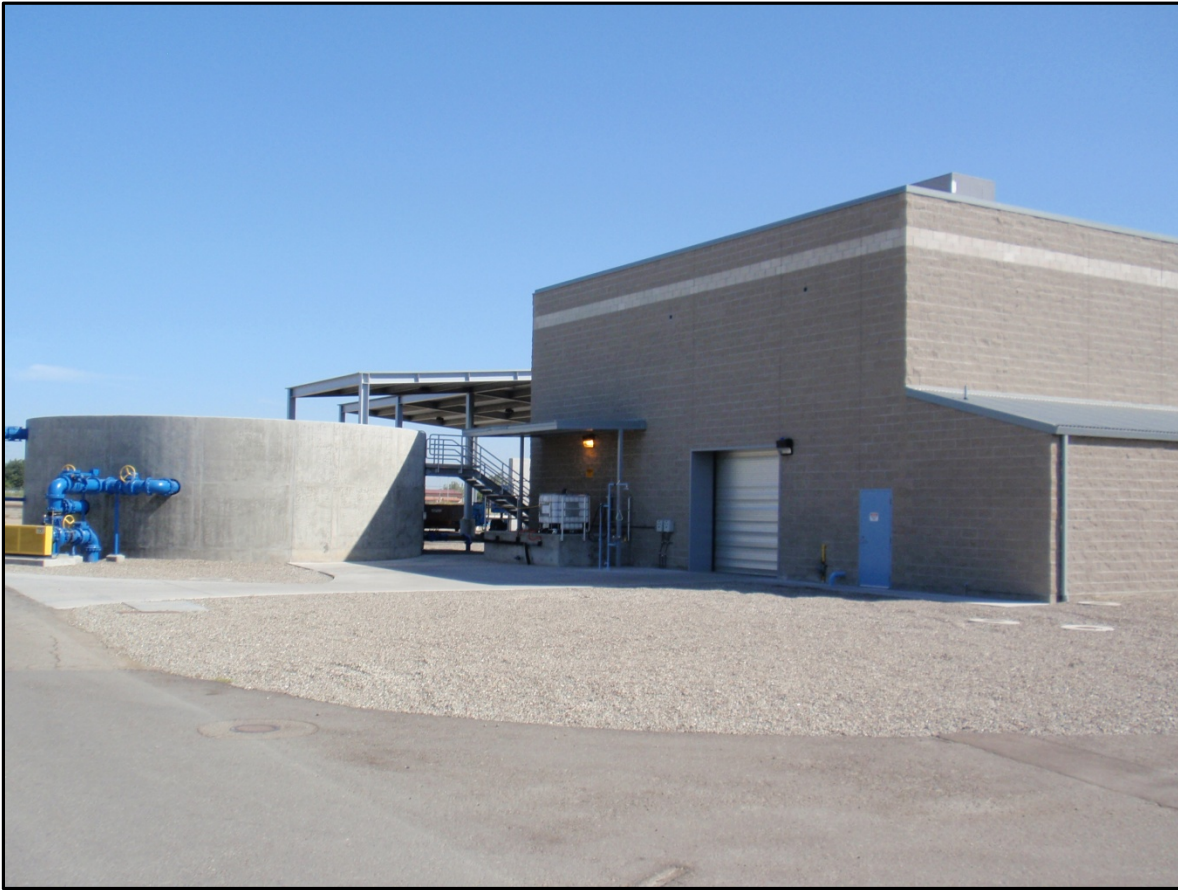
Figure 6.5-1, Solids Holding Tank and Dewatering Building
